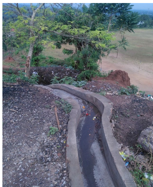
Figure 17: Rainwater drainage with waste
