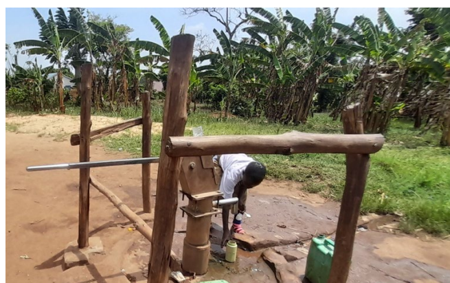
Figure 8: Water from a borehole with a pump
